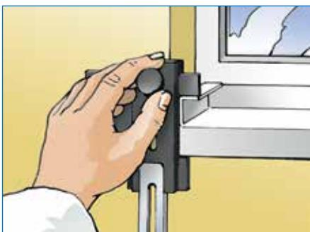
Moving the adjustment slider (D) to determine the upper edge of the windowsill as well as the overlapping of the insulating material and the edging profile of the windowsill.
