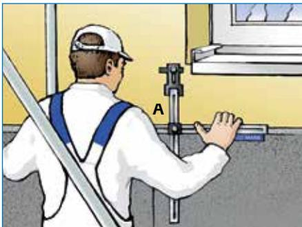
Place the horizontal stop (A) of the template on the previous insulation row when observing the prescribed plate offset.
