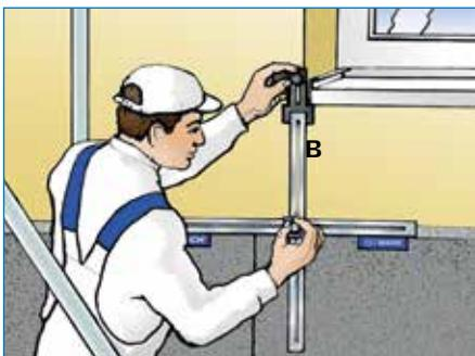
Moving the vertical stop (B) to the right until the windowsill and then upwards to determine the lower edge of the windowsill.
